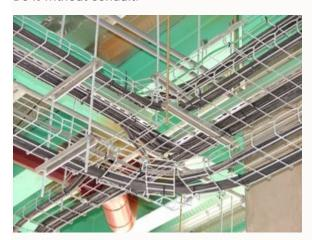
LAPP's TC-ER rated cables allow you to run cable outside of the tray without requiring a protective conduit, as long as the cable is secured every 6 feet.
